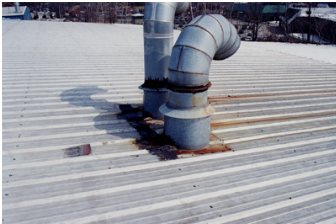
Stack Penetrations through old metal roof system
