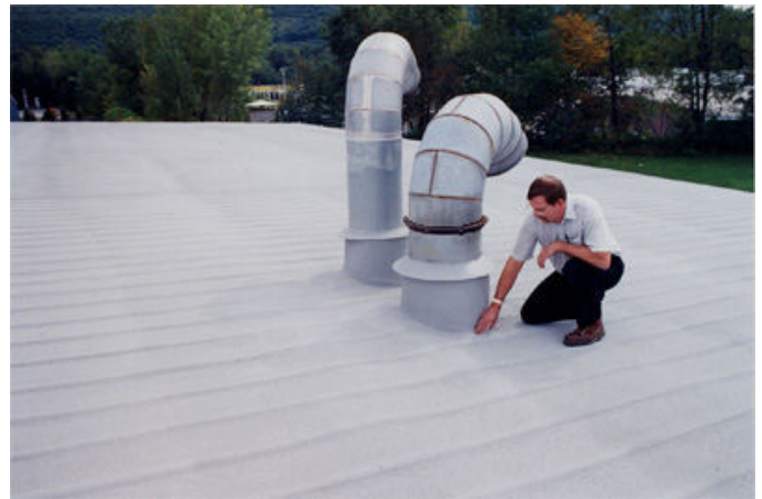
Stack Penetrations with new Seamless Spray-Foam roof system
