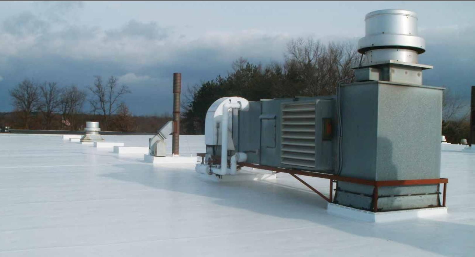
Minder knew that the design of a building's roofing system, particularly the amount of insulation used in the roofing assembly, could dramatically lower the building's energy use, as well as its energy bills. Reduced energy consumption would obviously be great for both the environment and the building owner's bottom line. While an insulation-free coating system was originally considered, Minder knew the best choice was a more energy-efficient system.
