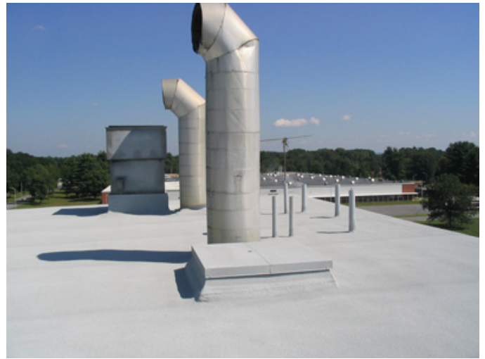
New Seamless, Self-Flashing Spray-Foam roof system
