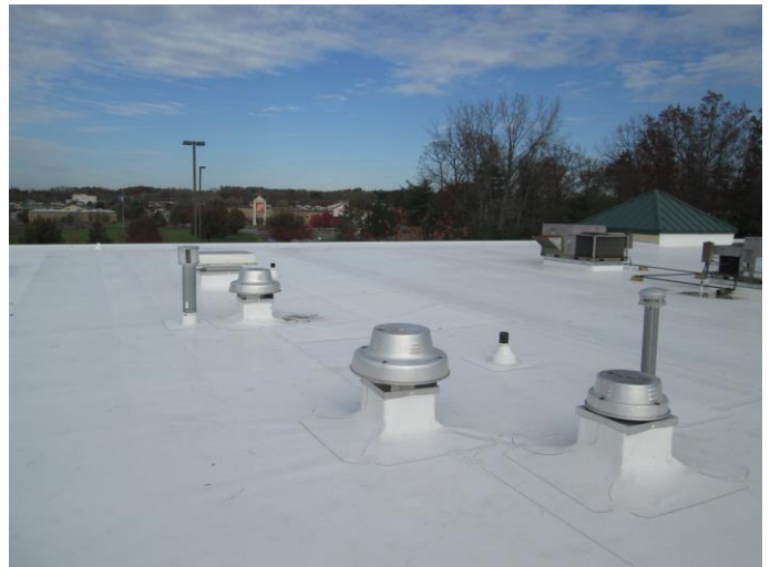
Newly installed 60 Mil TPO roof system
