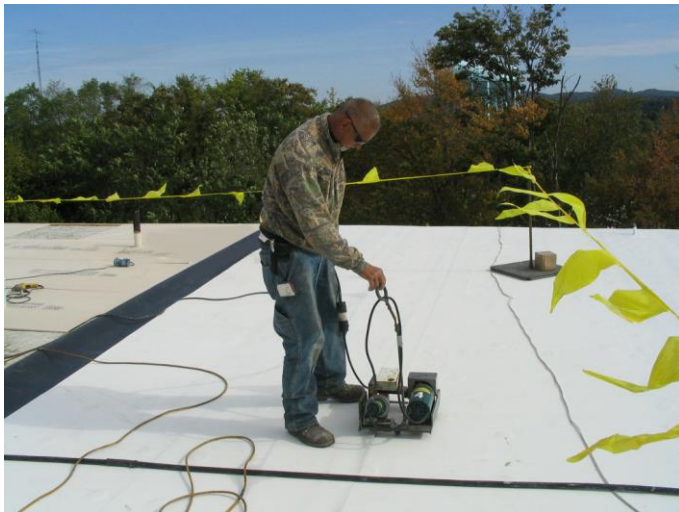
Hot-Air Welding TPO membrane seams
