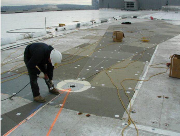
Installation of Tapered Insulation Crickets Between Drains
