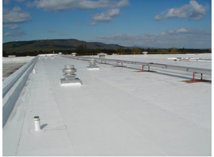
New Heat-Welded TPO Reinforced Roof Membrane
