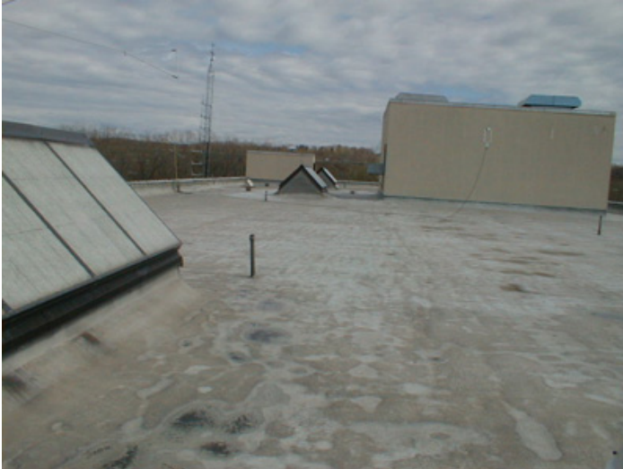
Old 1984 Spray-Foam roof system
