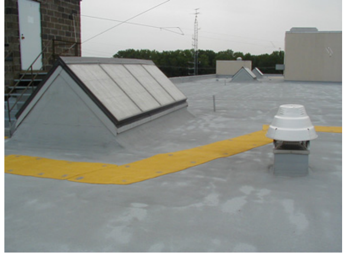
Spray-Foam roof with new Silicone Coating and Granules
