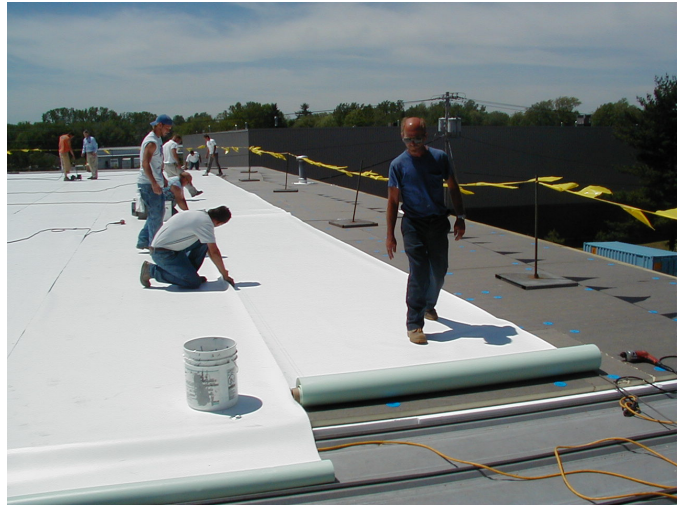
Crew positioning TPO membrane over new insulation
