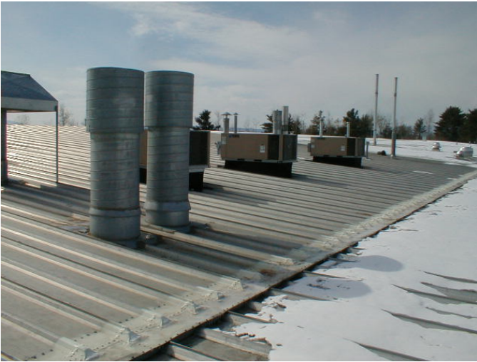
Old standing-seam metal roof
